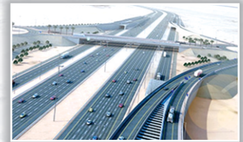
Dholera 10 Lane Expressway
