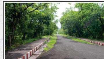
INTERNAL ROAD & PLANTATION
